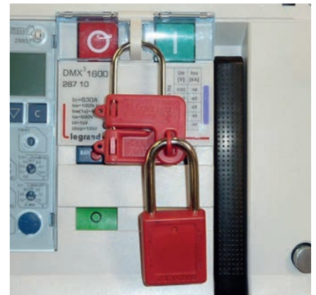
Padlocking the ON and OFF buttons
