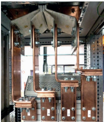
Kit for connection between a draw-out DMX 3 size 2500 and an incoming SCP
