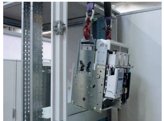
Placement of a fixed DMX 3
