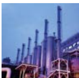
Category C3/C4 chemical industries
