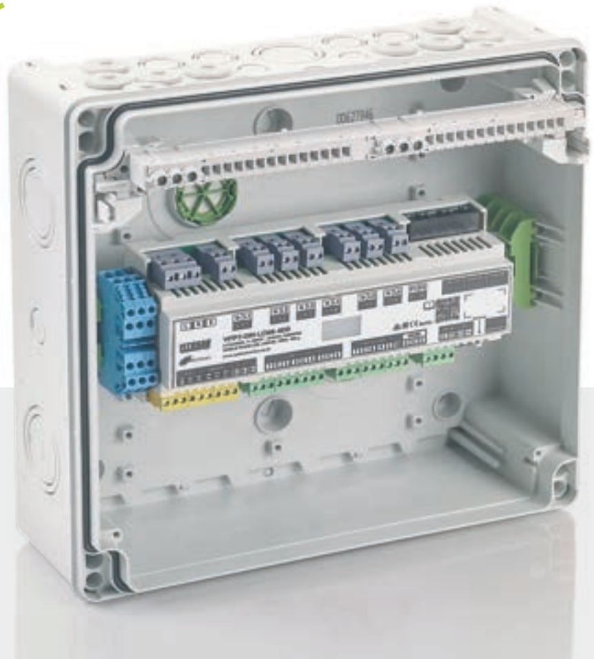
The compact installer-friendly housing is IP65 rated.
